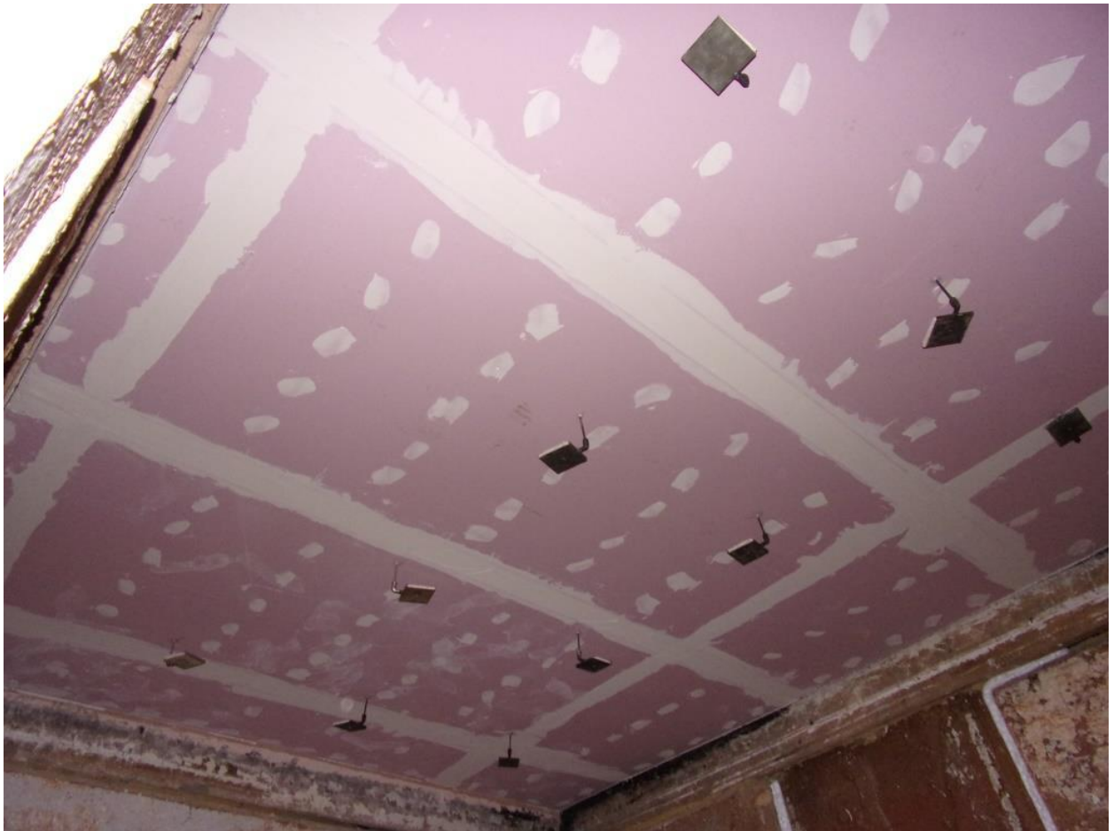
Exposed face of floor before test.
