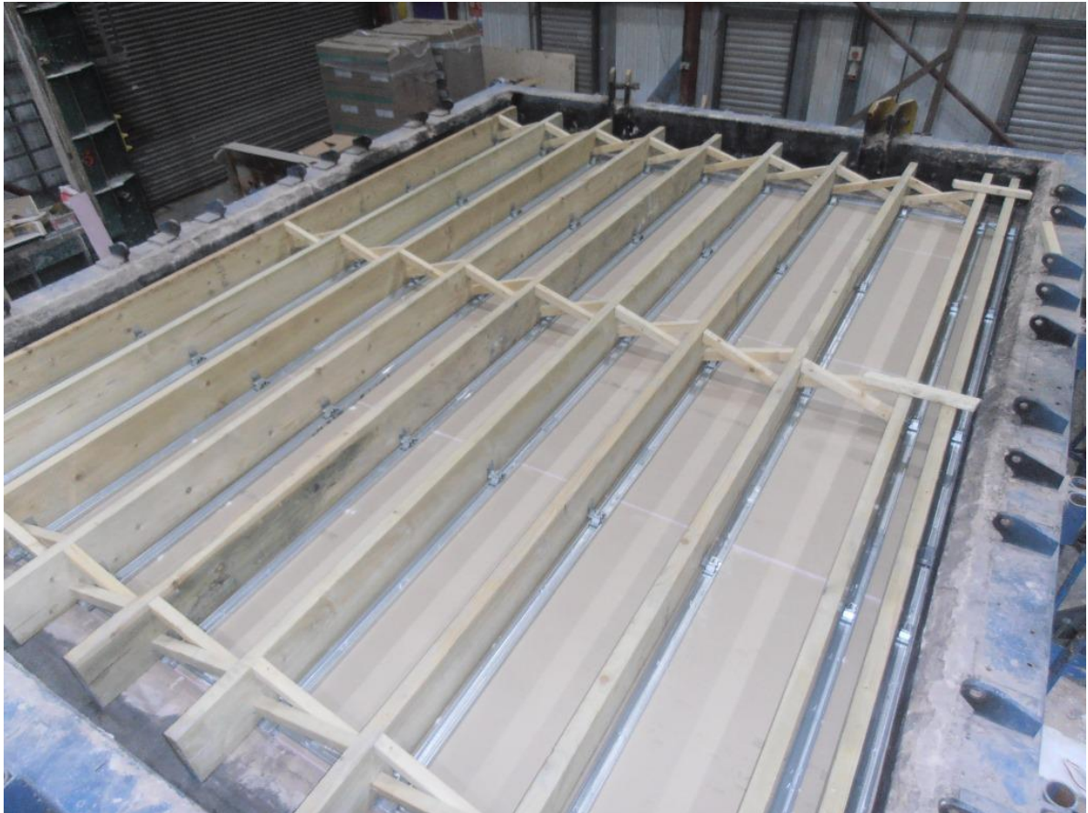
Floor during construction.
